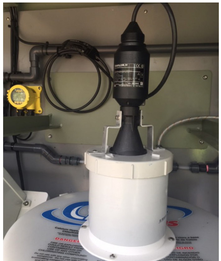
Level Measure Sensor to monitor briquette levels
